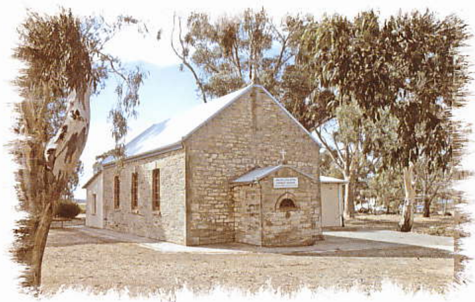
Polish Hill River Church after restoration
